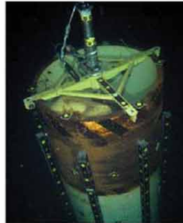
Pin pile with Transponder and photo targets
