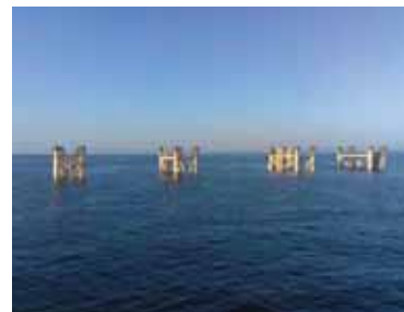
DUQ and PCWU jackets in Position and Docked onto the Pin Piles.
