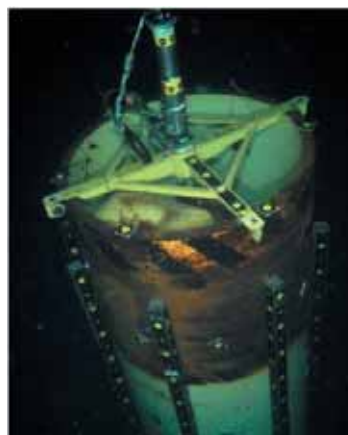
Pin pile with Transponder and photo targets
