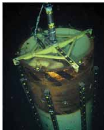
Pin pile with Transponder and photo targets
