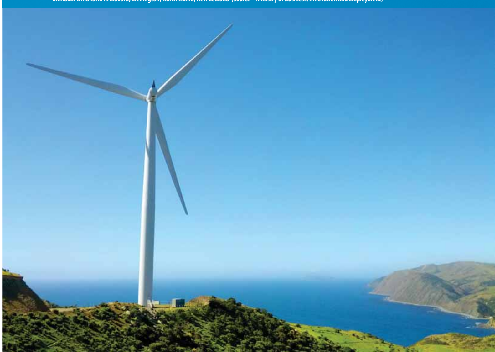
Meridian wind farm in Makara, Wellington, North Island, New Zealand (Source – Ministry of Business, Innovation and Employment)
