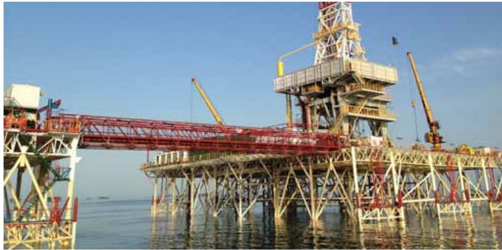
tonnes of condensate, can be assessed as a grandiose achievement of the Complex Drilling Works Trust. The management of SOCAR took part in this ceremony that coincided with the commencement of drilling operations. A ten block jacket, designed for drilling of three production wells, was installed at a depth of 26m of the sea. The most advanced technical and technological achievements, applied in the field of global drilling, were used while drilling the well #124.
