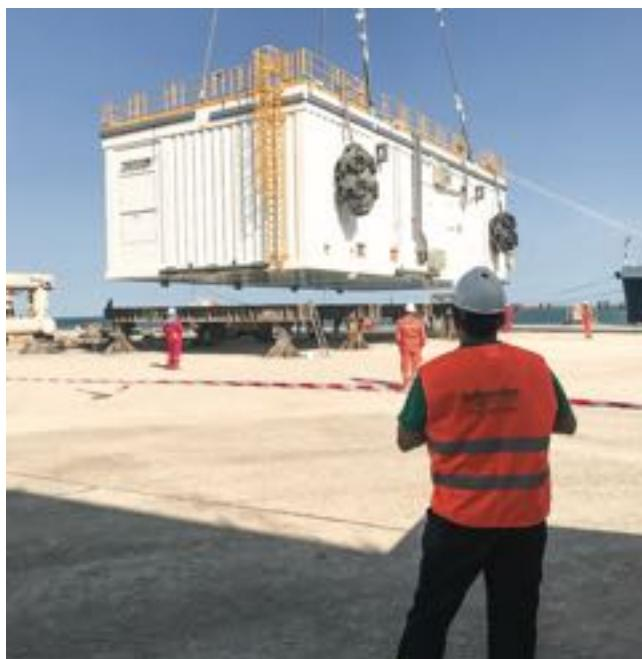
Schneider Electric is providing a range of technologies that will power the offshore facilities at Absheron, Azerbaijan's latest gas field. The solution, called "E-House", will combine power and control equipment together in a compact design for safe and reliable electricity supply and was delivered in August 2021.
